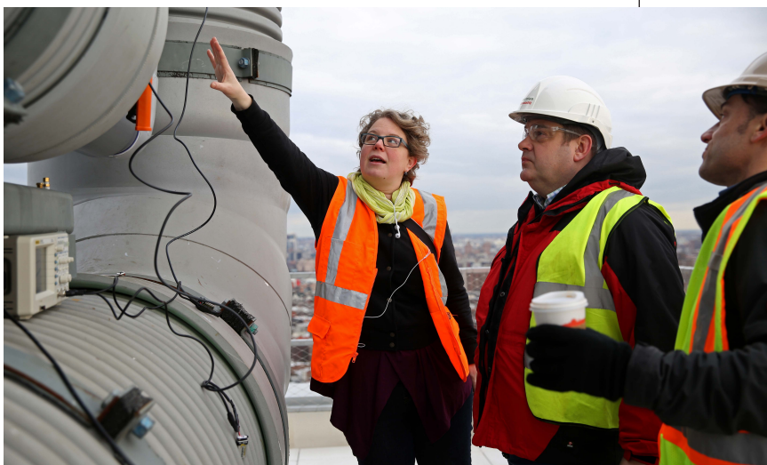
Elisabeth Malsch examines the first installation of Hummingbird, a fluid harmonic damper derived from NASA technology. Photo courtesy of Thornton Tomasetti.
